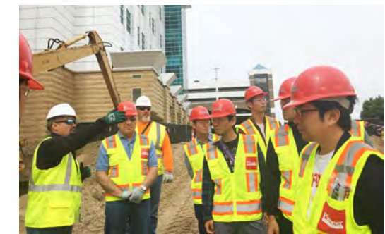
Construction Site Visit in Downtown Grand Rapids
