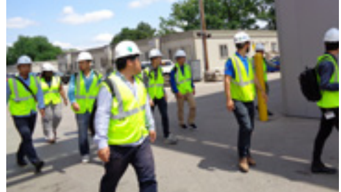
On a constructiob site tour of the MSU FRIB (Facility for Rare Isotope Beams)
